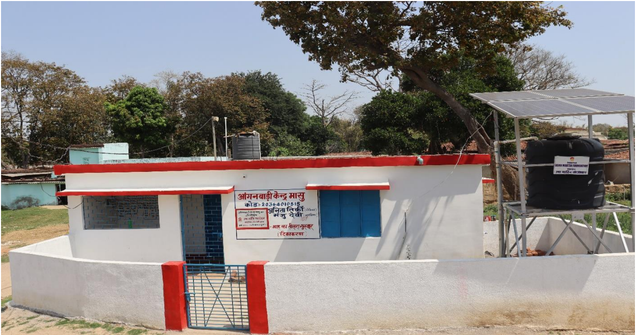
Photo—New construction of Masu Aganbari Kendra
