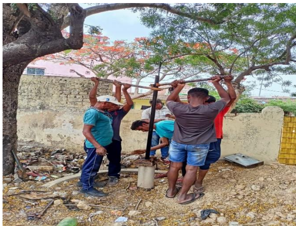
Hand pump repairing
