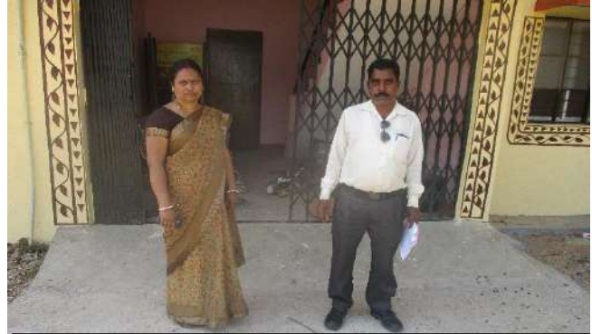
Repairing work and Soak pit Construction at Tati West Health Sub Center
