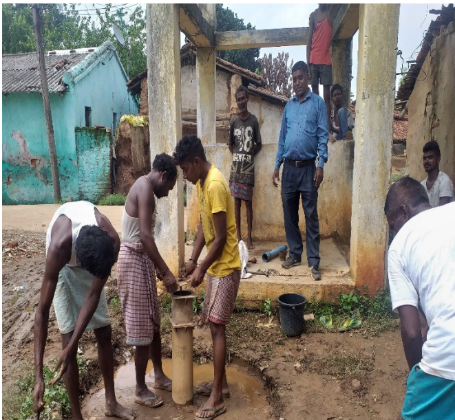
Figure- 2: Hand pump Repair at Haratu
